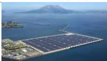
Figure 1a: The 'Floating' solar power plant in Kagoshima Bay, Japan can be considered as good example for saving space and the panels over water have a cooler temperature, which makes them more efficient. Finally the blue colour of the panels matches with the blue of the water which means that they do not disturb aesthetically. (Photo: © KYOCERA Corporation)
