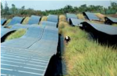
Figure 43d. Type b) Agrinerie® (2.1 MWp), La Reunion (FR). It combines energy generation from PV and lemon grass production. This dual land use design pattern allowed the developers to get the approval for the realization of a system, since in French overseas islands it is not allowed to build on ground PV, because of land and landscape protection rules.
