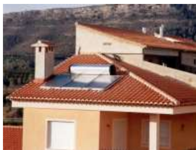
Figure 45a. Type a) Domestic Solar Hot Water System on the roof of a
