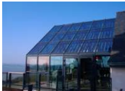
Figure 43b: Type a) Roof integrated photovoltaics. Glass-glass PV modules can be used in replacement of standard glazed surfaces (facades, roofs, skylights) in building's envelopes, coupled with standard framing systems. (Photo courtesy of Ertex Solar).
