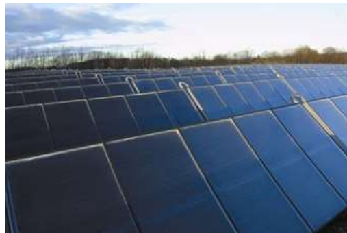
Figure 46c. Type b) Solar Thermal Collector field on the ground (Photo: ARCON/ESTIF, 2016)
