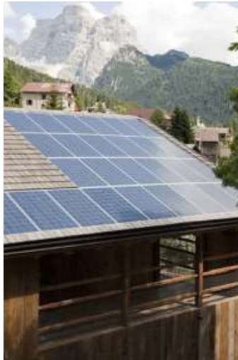
Figure 43a: Type a) Roof integrated photovoltaics, Tabià in Selva di Cadore (IT). Design Exit. Special BIPV opaque components (modules + framing system) replace the traditional wooden tiles of the roof. (Picture courtesy of Exit)
