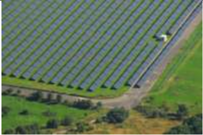
Figure 44c. Type b) Waldpolenz solarpark (40MW), Leipzig (DE). This PV system is a typical image for a large scale PV; it is built on a former military area. The modules are arranged in a parallel stripes pattern, are E_W oriented, and they face the South with an optimal tilt inclination of about 30°.
