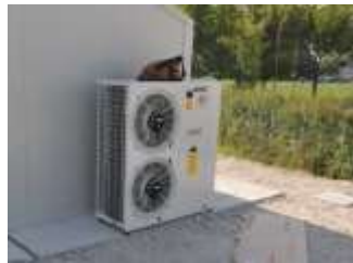
Figure 39a: Air source heat pump, Ferrara (Photo: M. Bottarelli, 2017)
