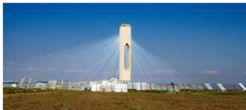
Figure 47. Solucar PS10 is the first solar thermal power plant based on tower in the world that generates electricity in a commercial way, 2007 (Photo: © SOLUCAR PS10 (2)).
