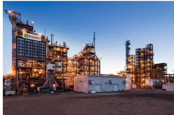
Figure 19d Full-scale biofuel facility in Edmonton, Canada. Publication permission by Enerkem (Source: http20 )
