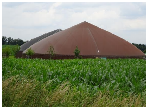
Figure 19c Bigger biogas plant on a farm in Oberscheid, Germany. (Photo: Alexandra Kruse 2016)
