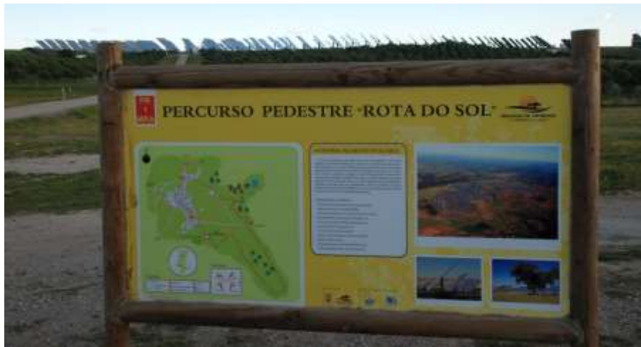
Figure 2. The Amareleja photovoltaic solar power plant visited by the COST TU1401 RELY (Renewable Energy and Landscape Quality) participants on the 25 th of March, 2015
