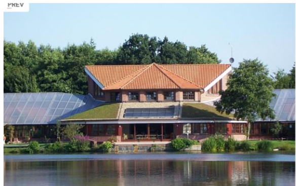
Figure 34b: Historic-Ecological Education Center Papenburg/Germany, built in 1988: Towards the North there are earth walls as energetic protection, towards the south a winter garden, which serves as semi-tropical greenhouse and as corridor between the accommodation units and common facilities. The bricks which store the temperature have been recycled. (Photo: http43 )
