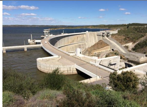
Figure 23b Large hydro power plant Alqueva II in Portugal. (Photo: Naja Marot 2015)
