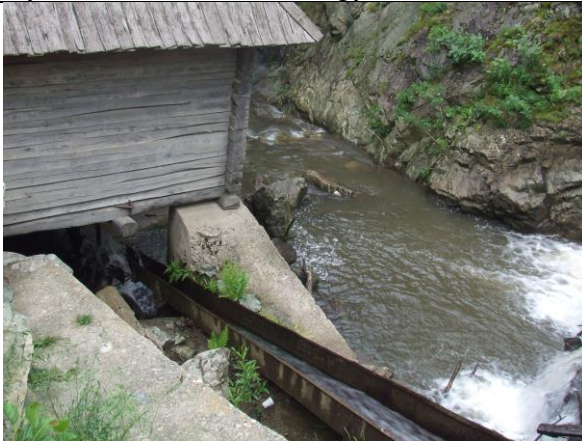
Figure 23a Micro hydro power in Eftimie Murgu village, Caraş Severin county, Romania. (Photo: Maria Bostenaru Dan 2008)
