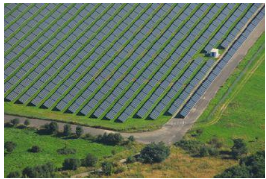
Figure 25c Type b) Waldpolenz solarpark (40MW), Leipzig (DE). This PV system is a typical example of a large scale PV; it is built on a former military area. The modules are arranged in a parallel stripes pattern, are E-W oriented, and face the South with an optimal tilt inclination of about 30°. (Photo : Juwi Solar GmbH)
