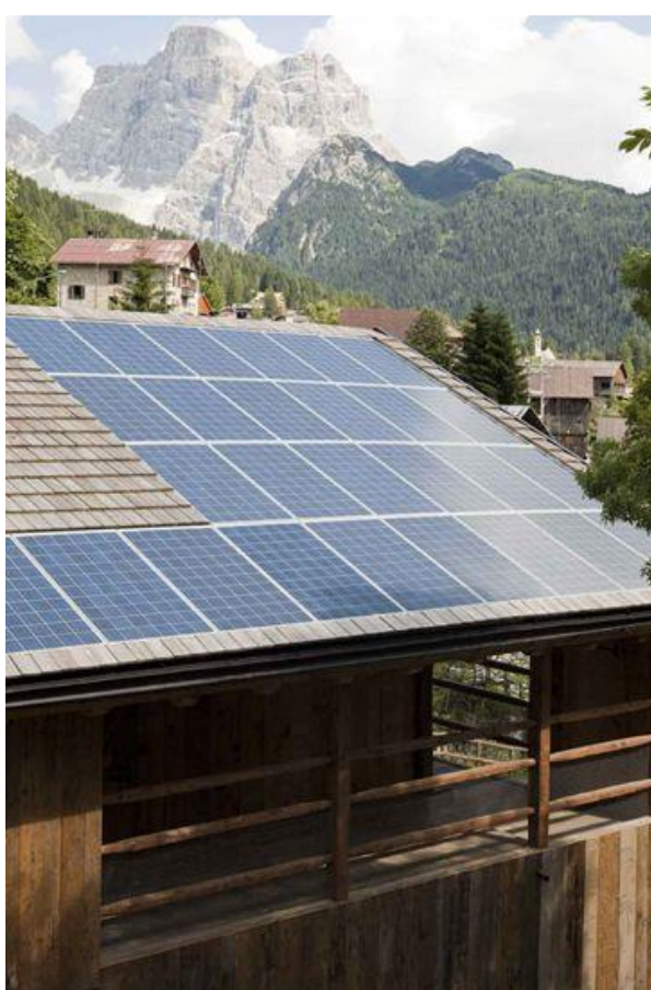
Figure 25a Type a) Roof integrated photovoltaics, Tabià in Selva di Cadore (IT), designed by Exit. Special BIPV opaque components (modules + framing system) replace the traditional wooden tiles of the roof. (Photo courtesy of Exit)
